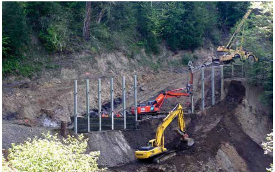
Construction of Soldier Pile Wall
