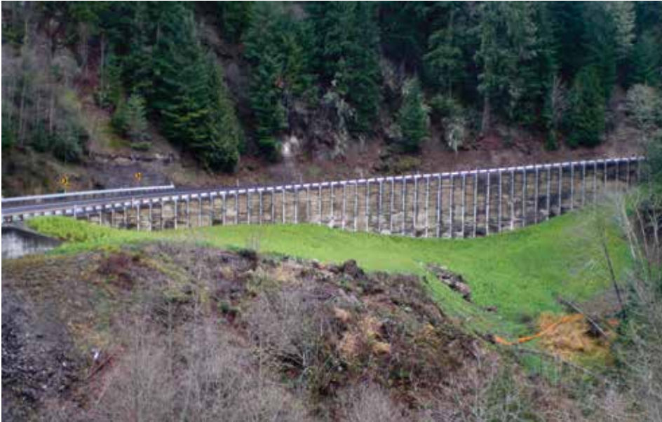
Completed Ground Stabilization Wall
